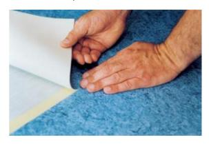
Clean the seam area and fix a **special**, even masking tape (article no. 50000), which is resistant against our cold-welding liquid, centred over the closely cut seam. This is absolutely necessary to avoid damage to the floor finish (e.g. made of Polyurethane) of the floor covering.
