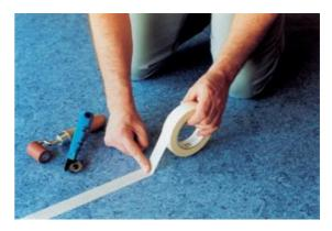
Press the **special** masking tape firmly to the PVC-floor covering by using a seam roll (article no. 50020), ensuring that no cold-welding liquid penetrates beneath the masking tape.
