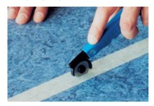
In case of hard and little flexible PVC-floor coverings (for instance Commercial Floor Coverings) warming up the seam area (to a maximum of 40 °C by using a blow dryer or an iron) before welding enables an easier and more even guidance of the needle in the seam.
