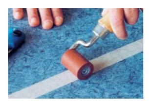
Easily cut the masking tape with the rolling knife (article no. 50010) in the seam area. Alternatively a straight blade or a hook-blade can be used. It is important not to damage the edges of the floor layers while cutting the tape. This can be done effectively by pressing the knife deeply into the seam, resulting in a good guidance.
