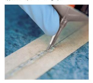
After about 10 minutes the cold-welding liquid on the masking tape is dry and the tape has to be removed steadily backwards at an angle. Swellings in the seam
